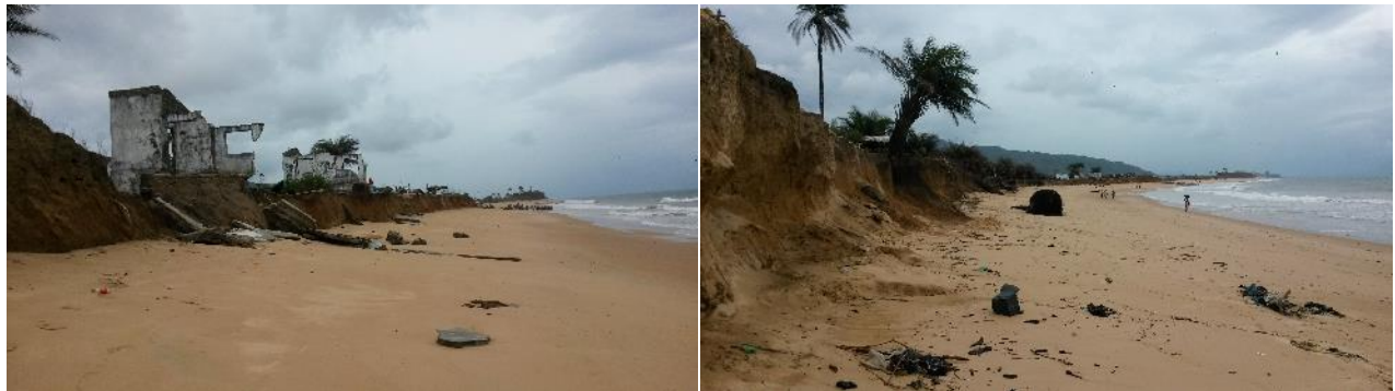
Plate 5. View of the degree of coastal zone retreat and eating up of infrastructures (left) and; Intensive beach erosion due to sand extraction and sea level rise (right) at Hamilton.
